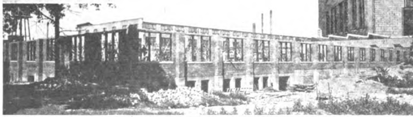
The Hudson Motor Car Co., Detroit, has increased its floor area by adding a third story to the main building (upper left) and also to three of the wings, the additions being shown in dark in the illustration
